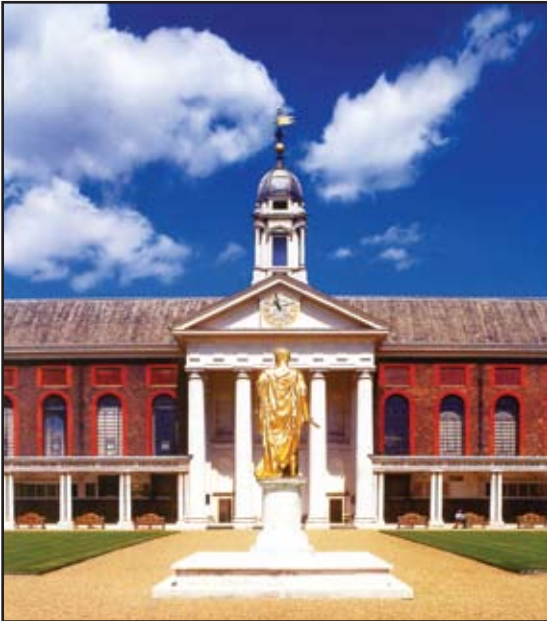
Figure Court with the gilded statue of Royal Hospital founder King Charles II. From the official guide, "The Royal Hospital Chelsea: The Royal Hospital Chelsea: The Place and the People."
