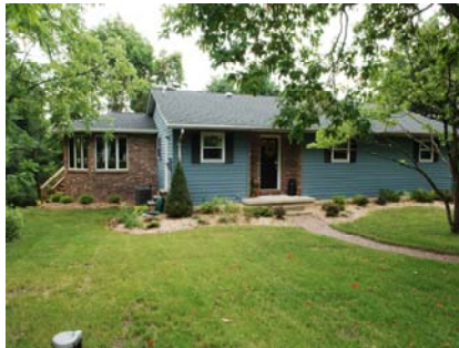
Addition Residential Construction Over $50,000. R.W. Buff, Inc.
