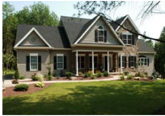
Residential Construction 2500-3000 sq ft R.W. Buff, Inc.
