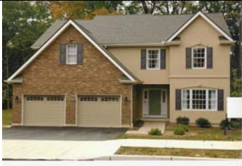
Residential Construction and Architecture 2000-2500 sq ft Buff-Nauman, Inc.
